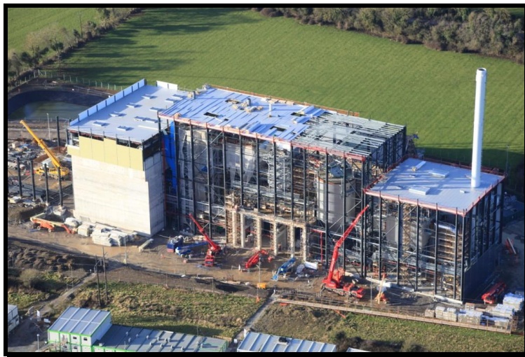
Aerial view of Meath waste-to-energy site – January 2011
